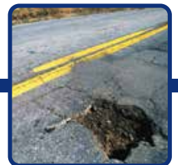
POTHoles/DAMAGED PAVEMENT
